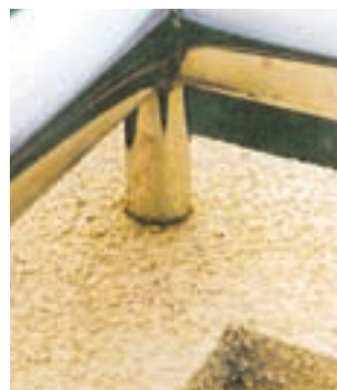
Common handrail detail where the handrail support penetrates the weather skin of the building and the top of the wall is not sloped to drain the water.
