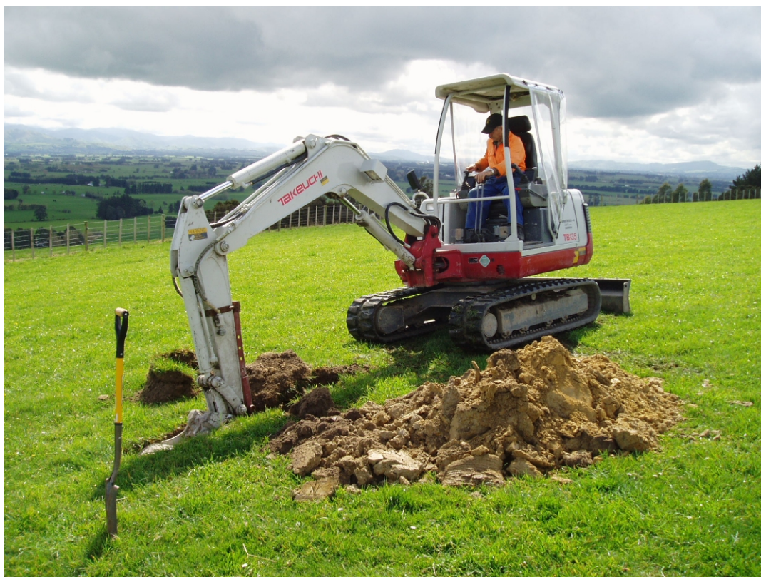
Photograph 2. Excavation of test pit 1
