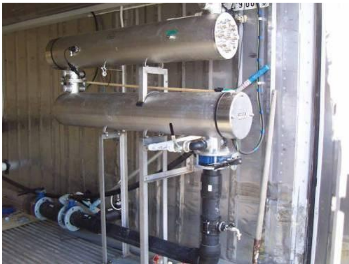
Figure 17. UV treatment reactors at the Carterton plant
