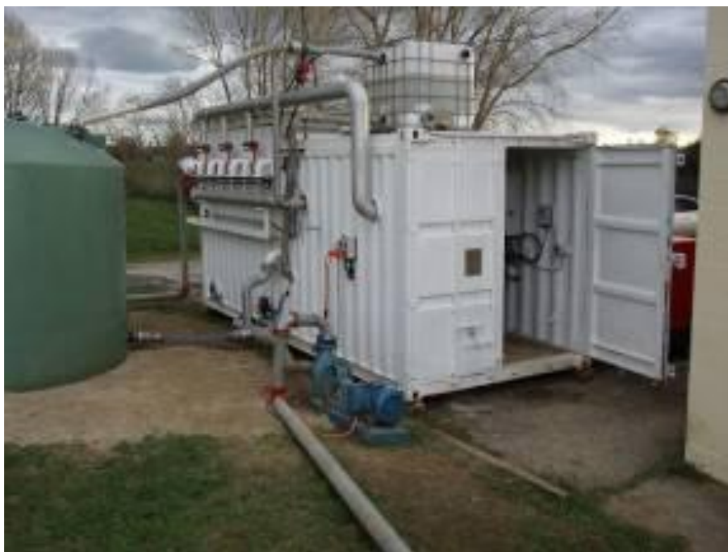
Figure 27. 900m 3 /day Membrane Plant.
