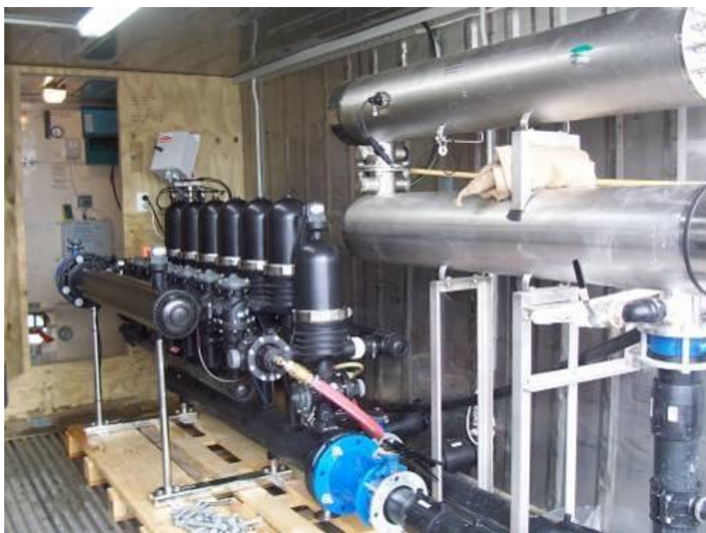
Figure 16. Existing Filtration Plant with the UV reactors in the foreground
